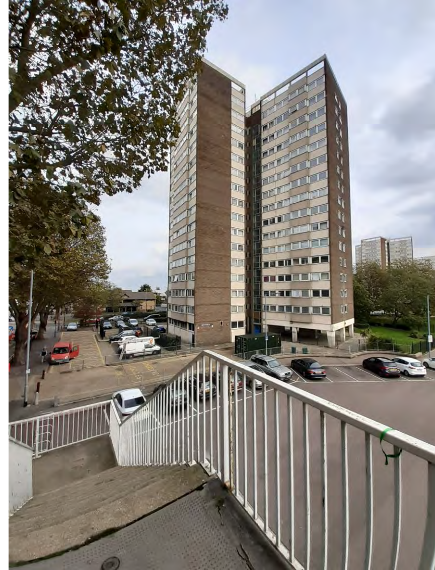
54. Quantock block seen from Chichester Road footbridge
