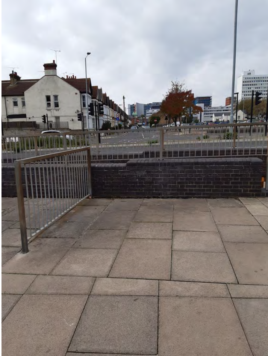
91. Queensway East side looking towards West across subway
