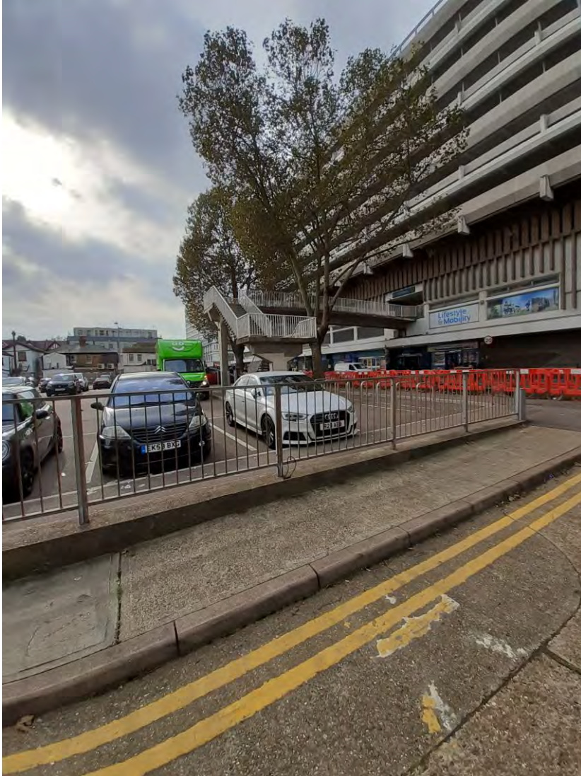
47. Looking South from Queensway towards Chichester Road with multi storey car park to right
