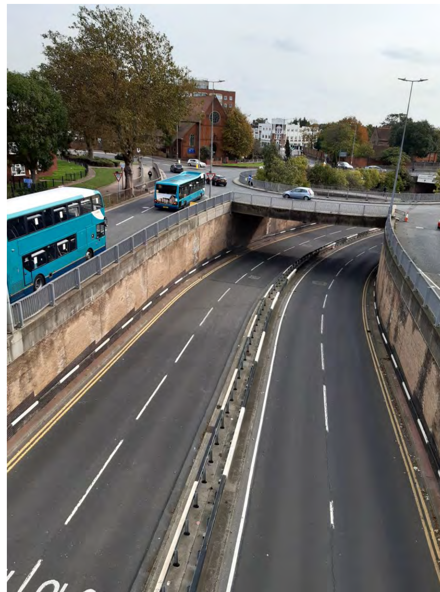
128. Queensway footbridge looking East into underpass
