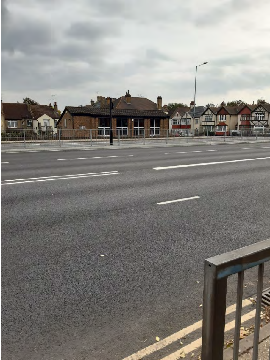
85. Queensway looking East from West Side of Road
