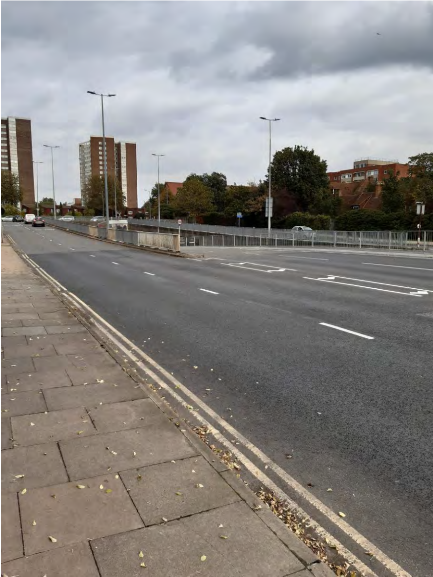
87. Queensway looking North towards underpass
