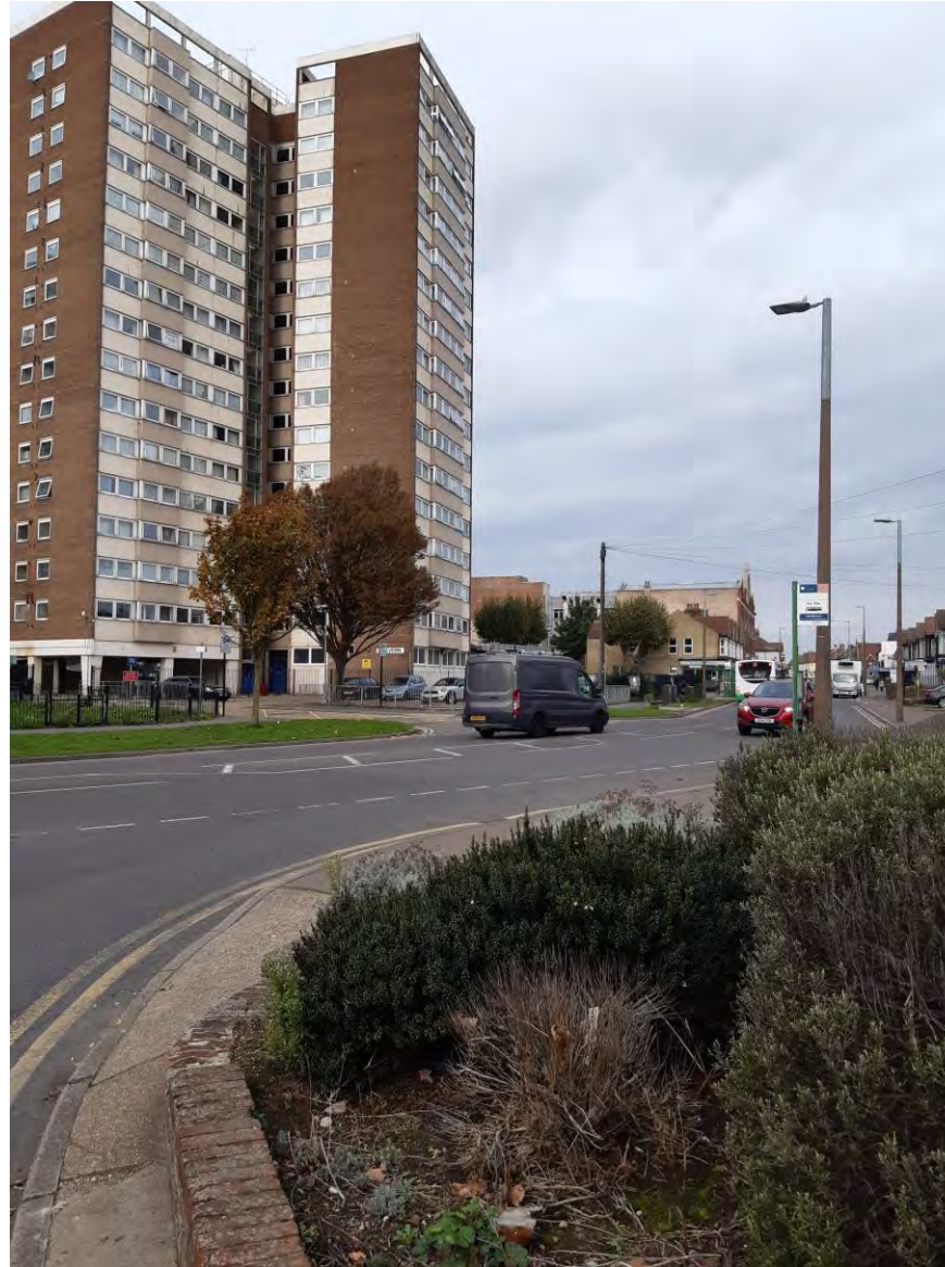
116. Looking North up Sutton Road towards Malvern Block
