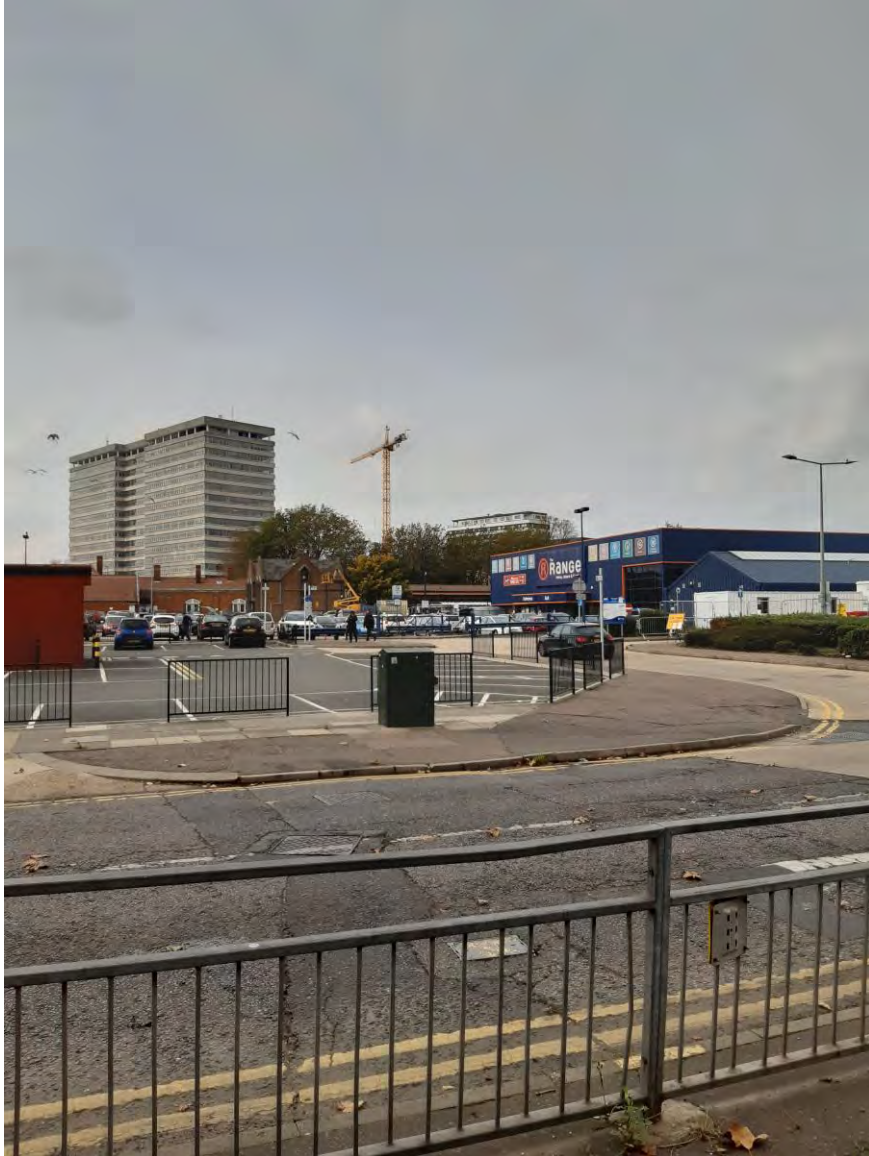
23. The Range site and Alexandra House in background
