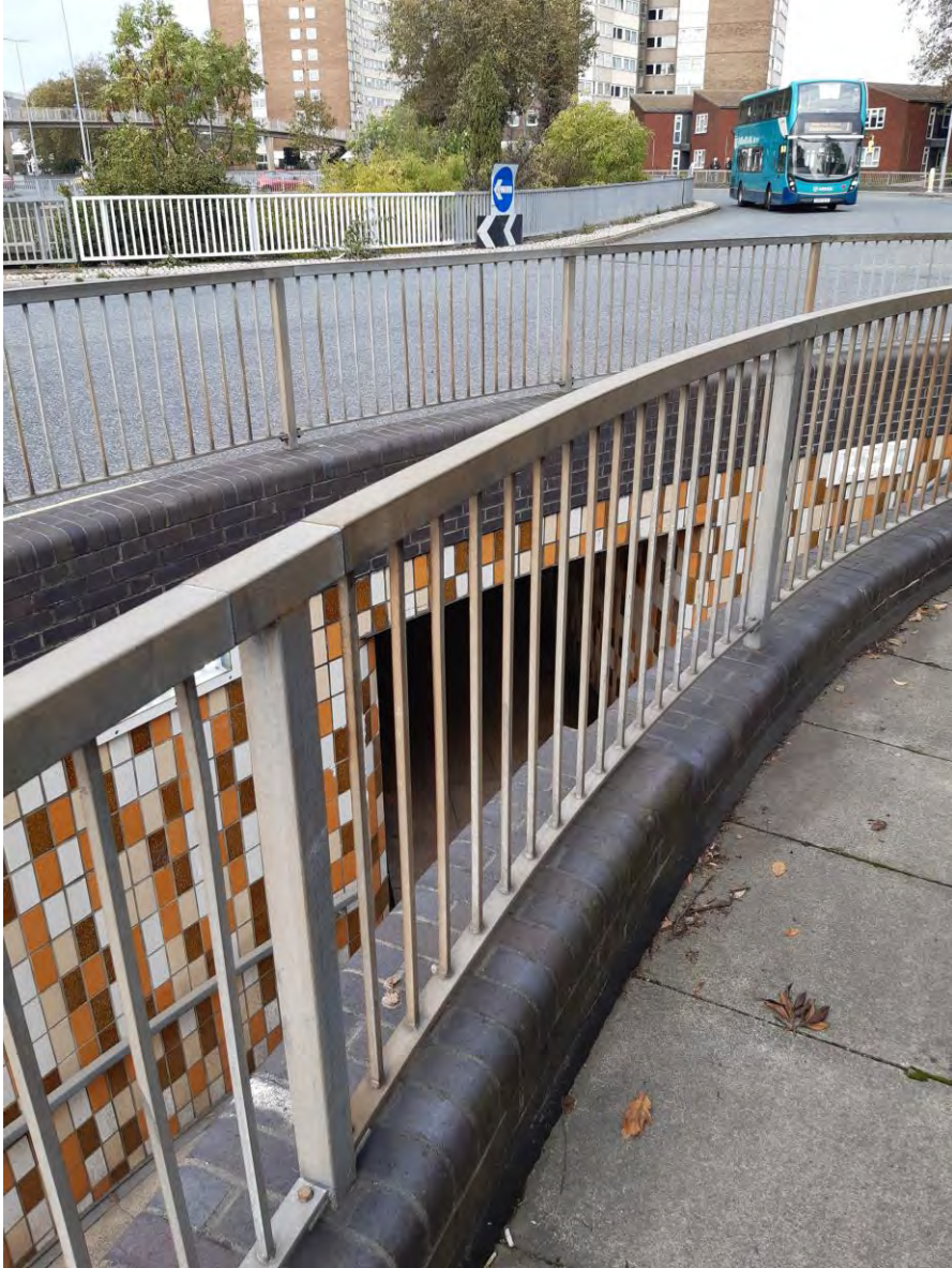
103. Queensway East side Roundabout subway entrance
