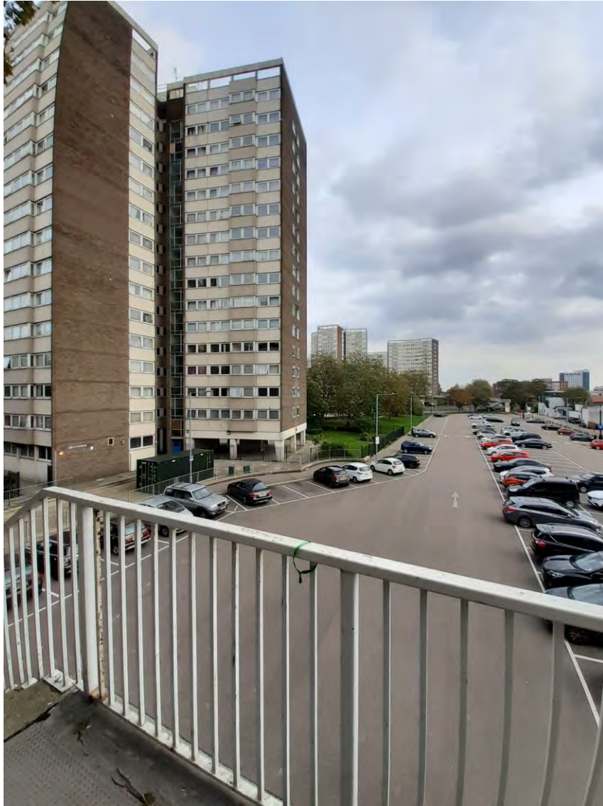
55. Quantock Block seen from Chichester Road footbridge
