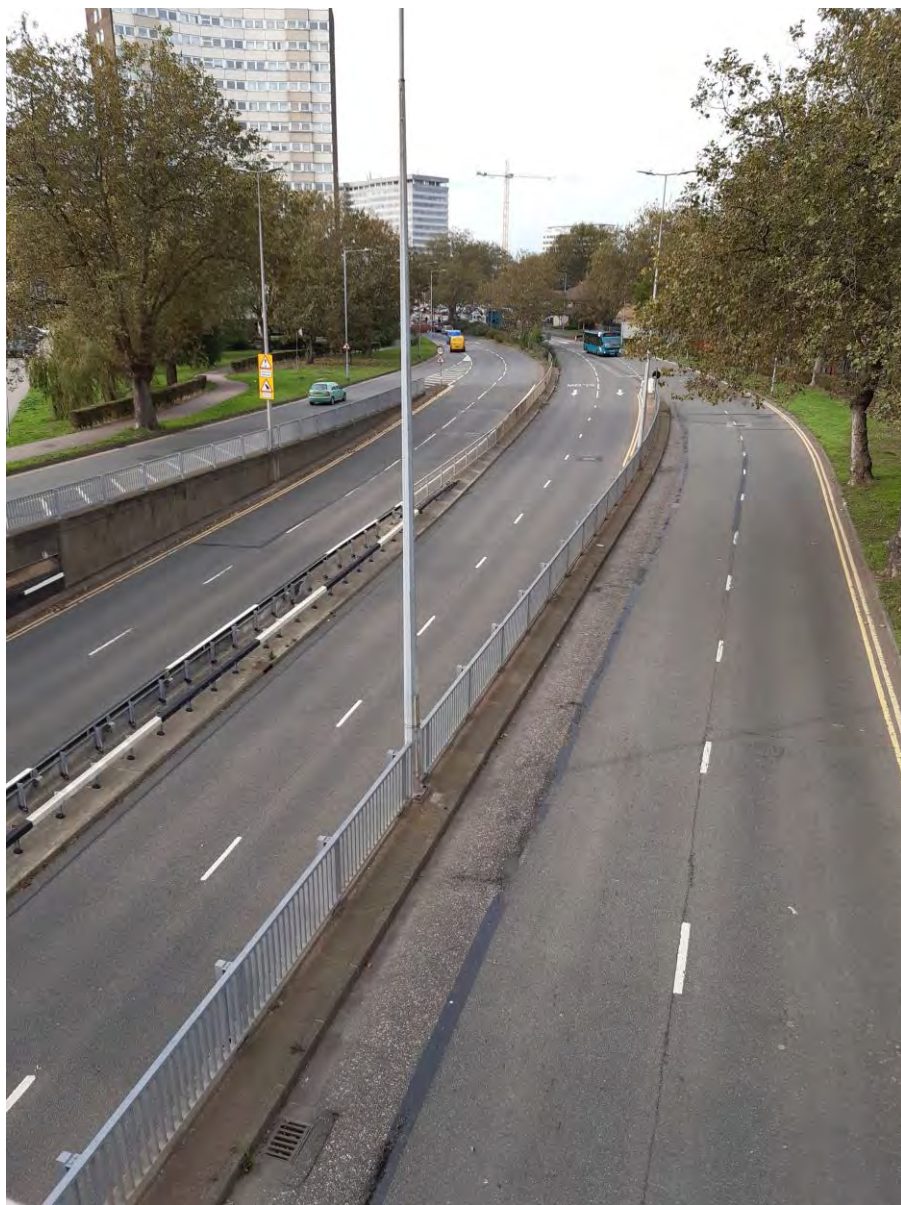
127. Queensway footbridge looking West
