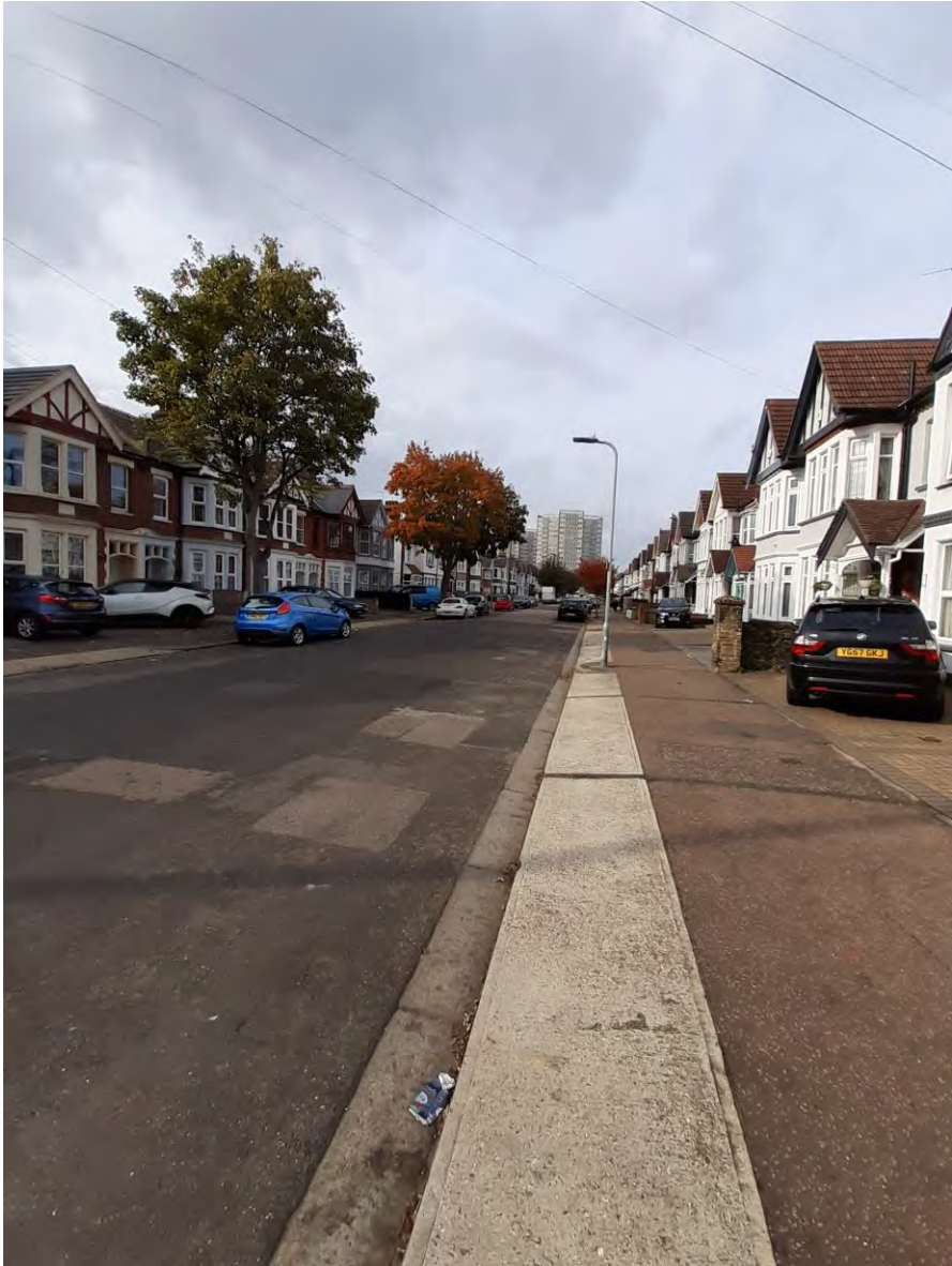
1. Boscombe Road looking West at existing blocks
