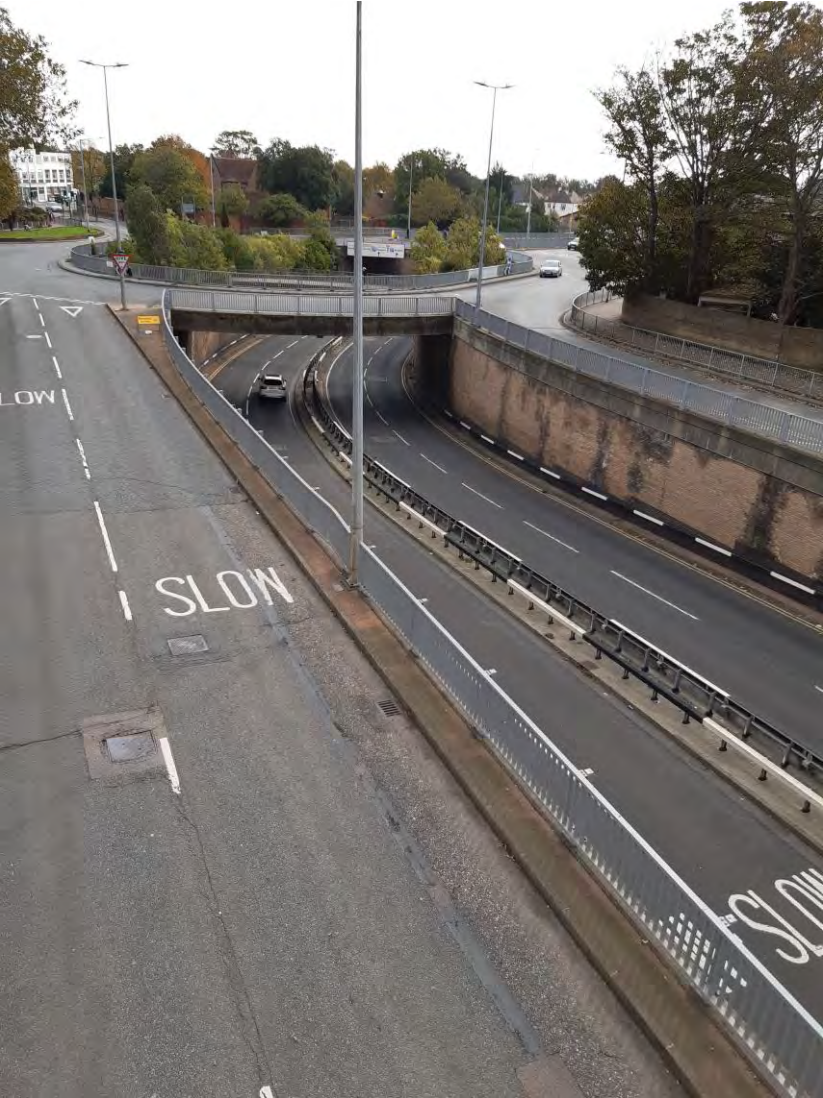
125. Queensway roundabout viewed from footbridge looking East
