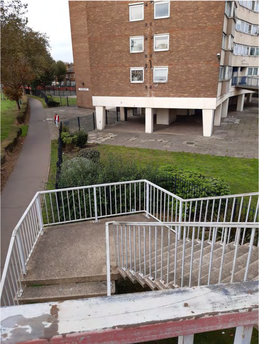
131. Queensway footbridge looking at Pennine block
