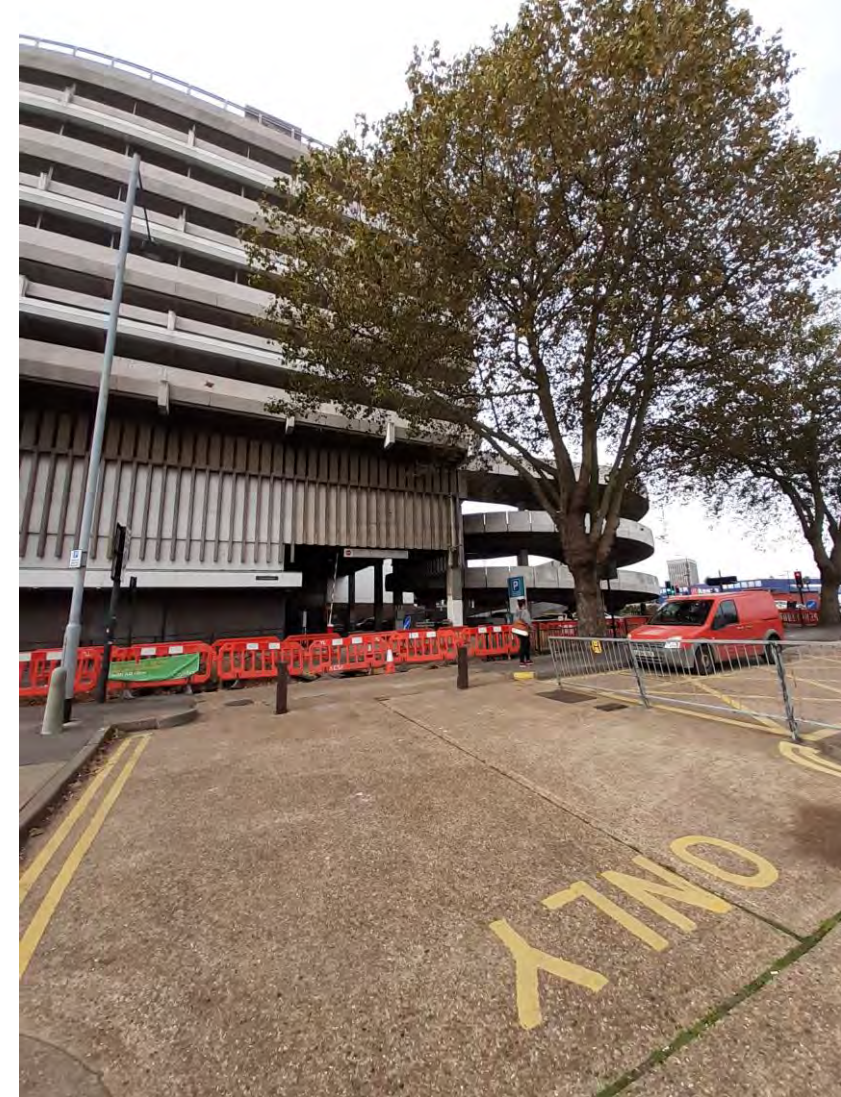
48. Looking West at multi storey car park
