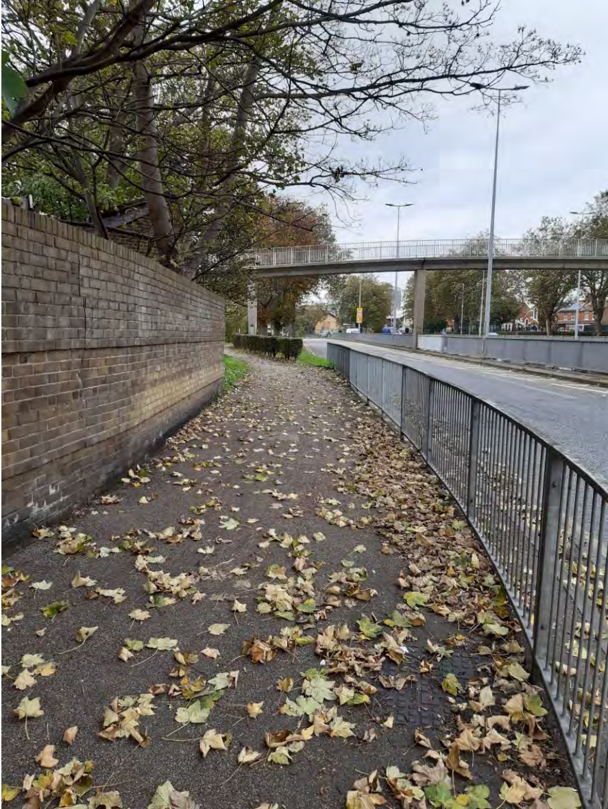
78. Queensway roundabout looking East towards Queensway footbridge
