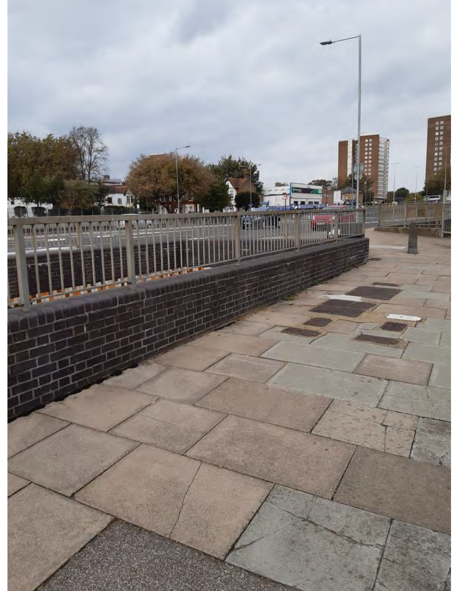
92. East side Queensway subway entrance
