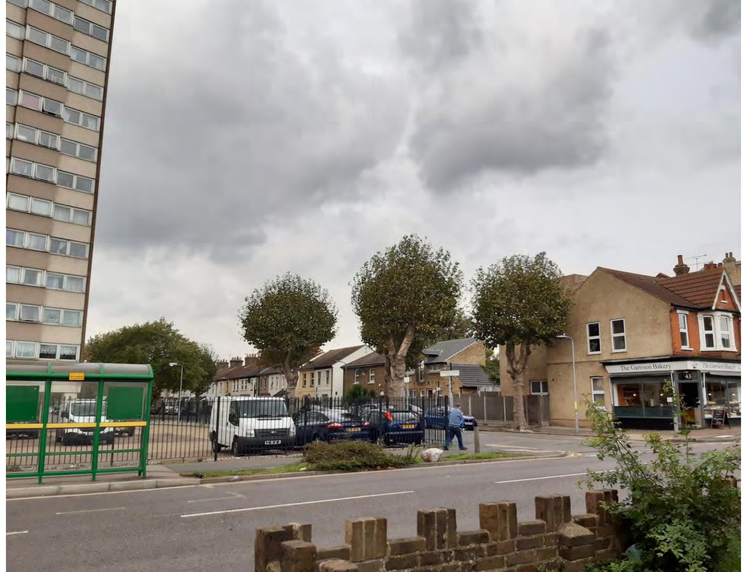
6. Malvern Block from Sutton Road looking towards Coleman Street
