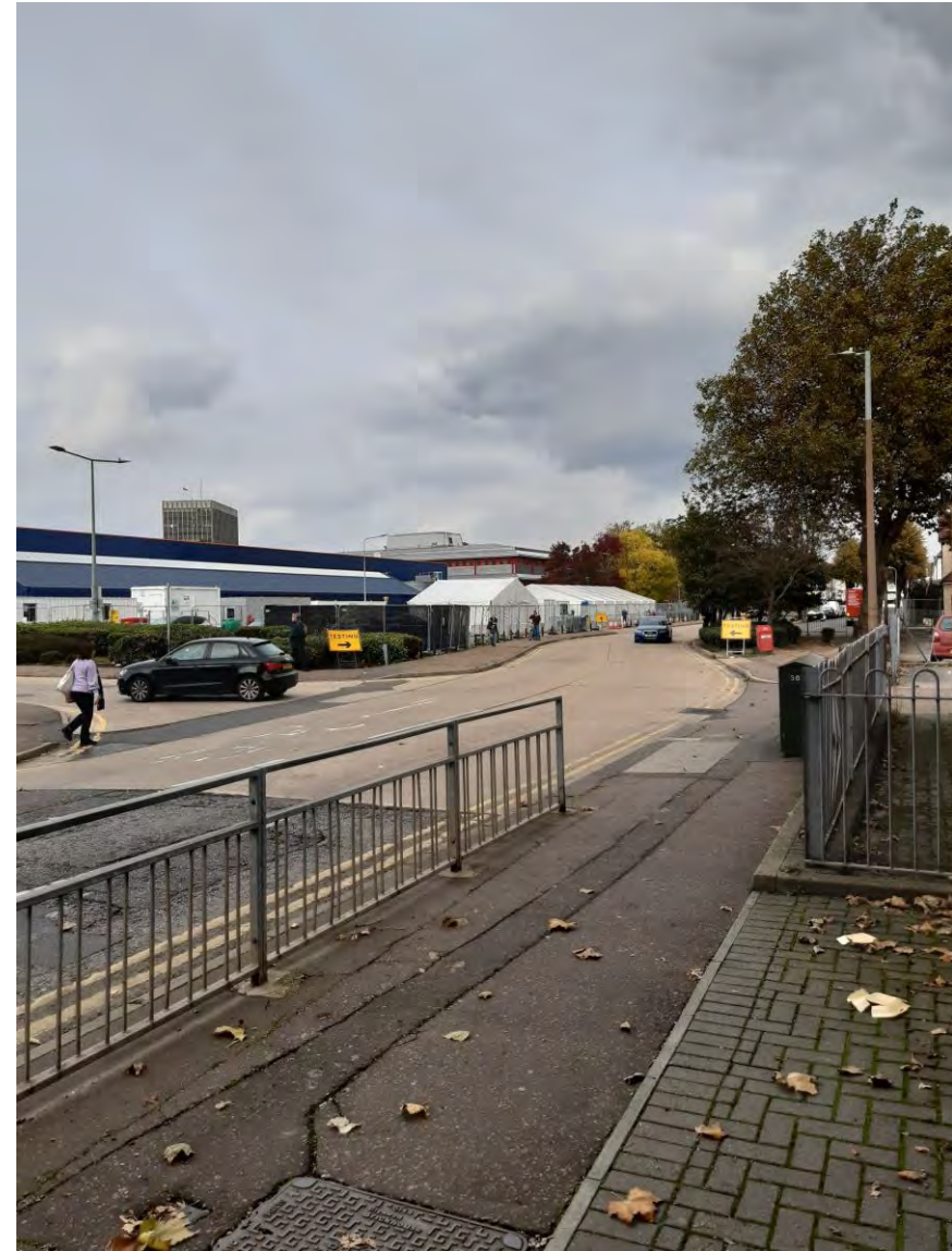
22. The Range site from junction of Queensway and Short Street
