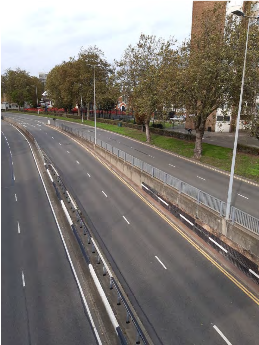
130. Queensway footbridge looking West
