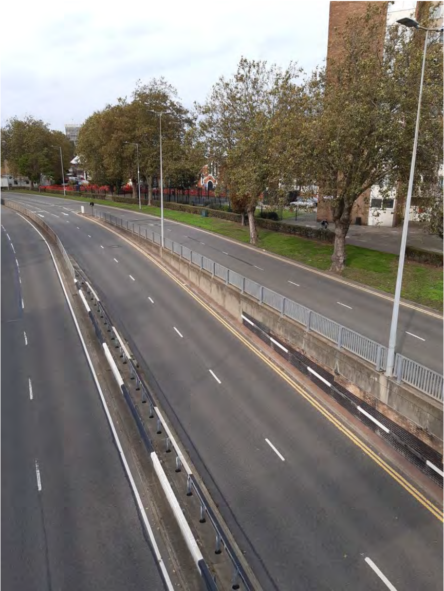
129. Queensway footbridge looking West
