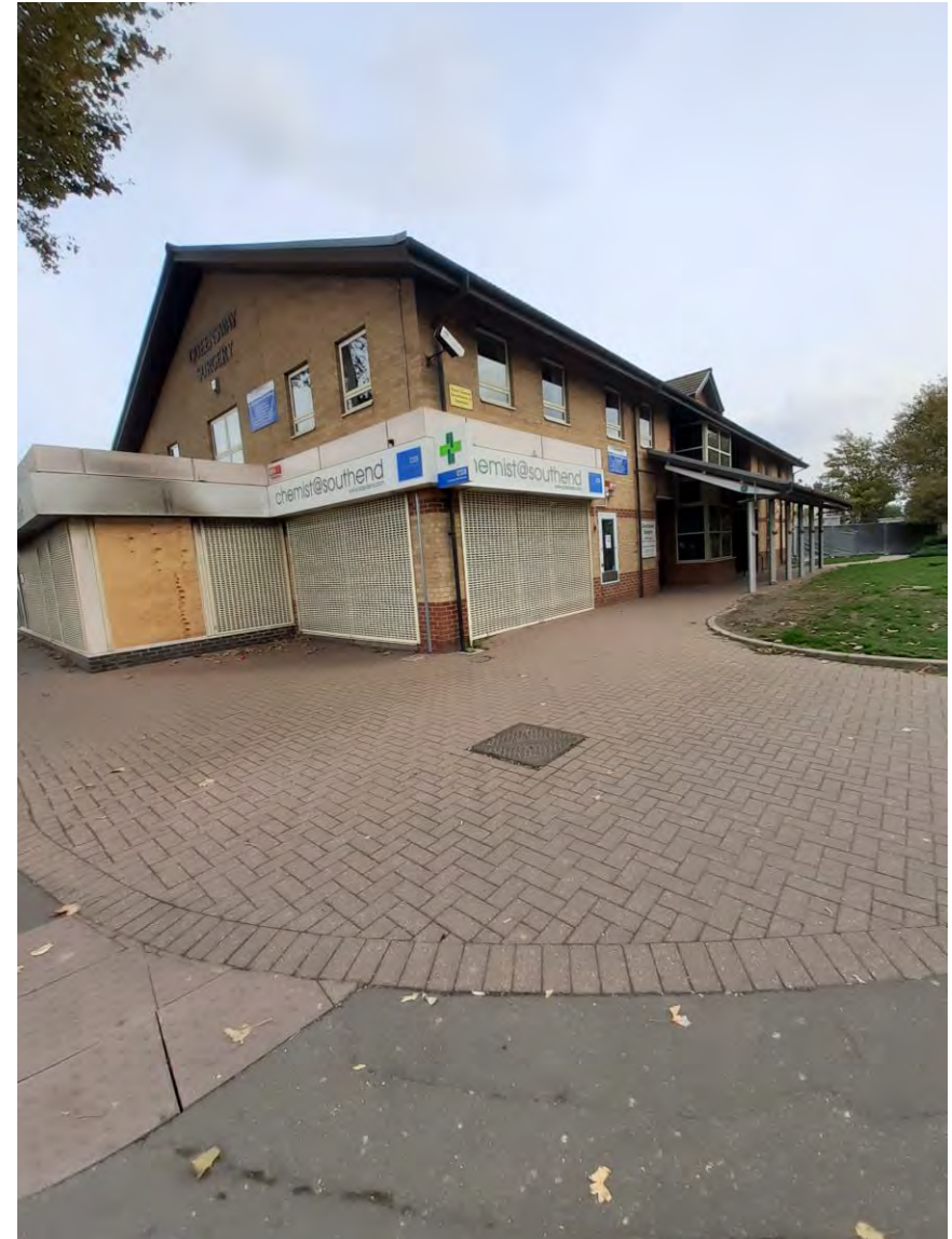
44. GP junction of Queensway and Short Street
