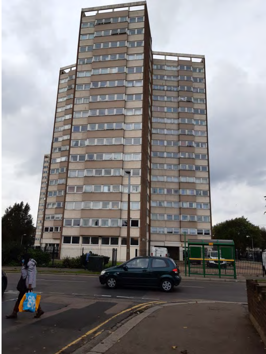
5. Malvern block view from Boscombe Road
